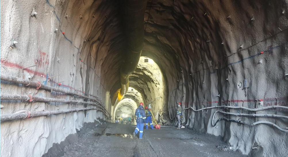
Katse TBM Access Adit
