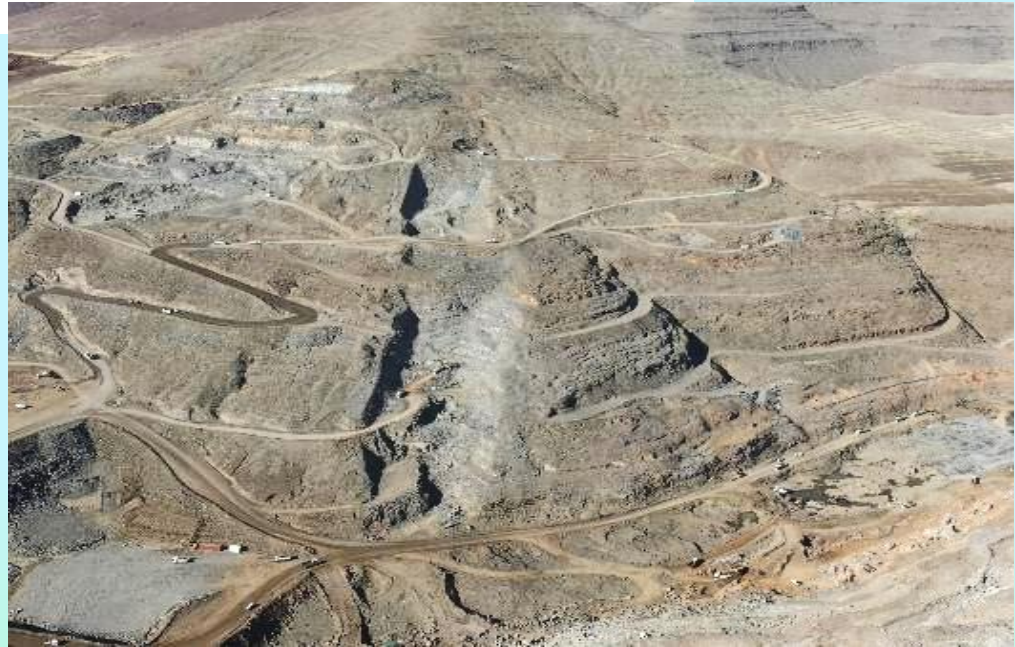
Left Bank Excavation
