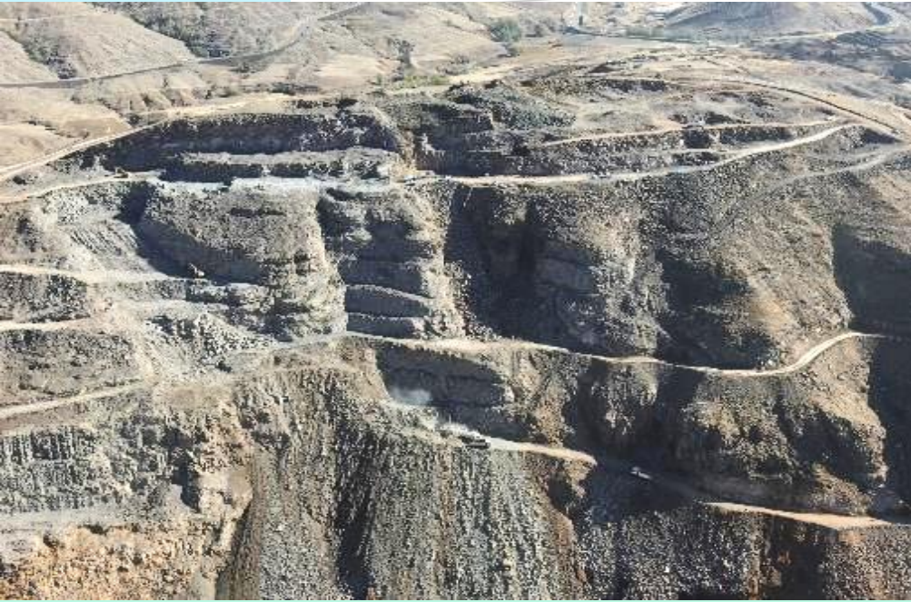
Main Dam Excavation: Right Bank
